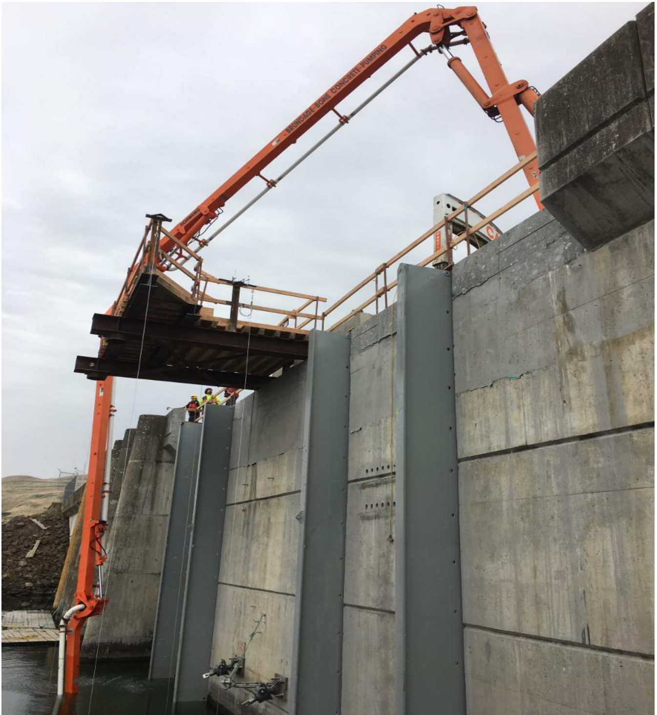
Pumping concrete for AWS intake structure
